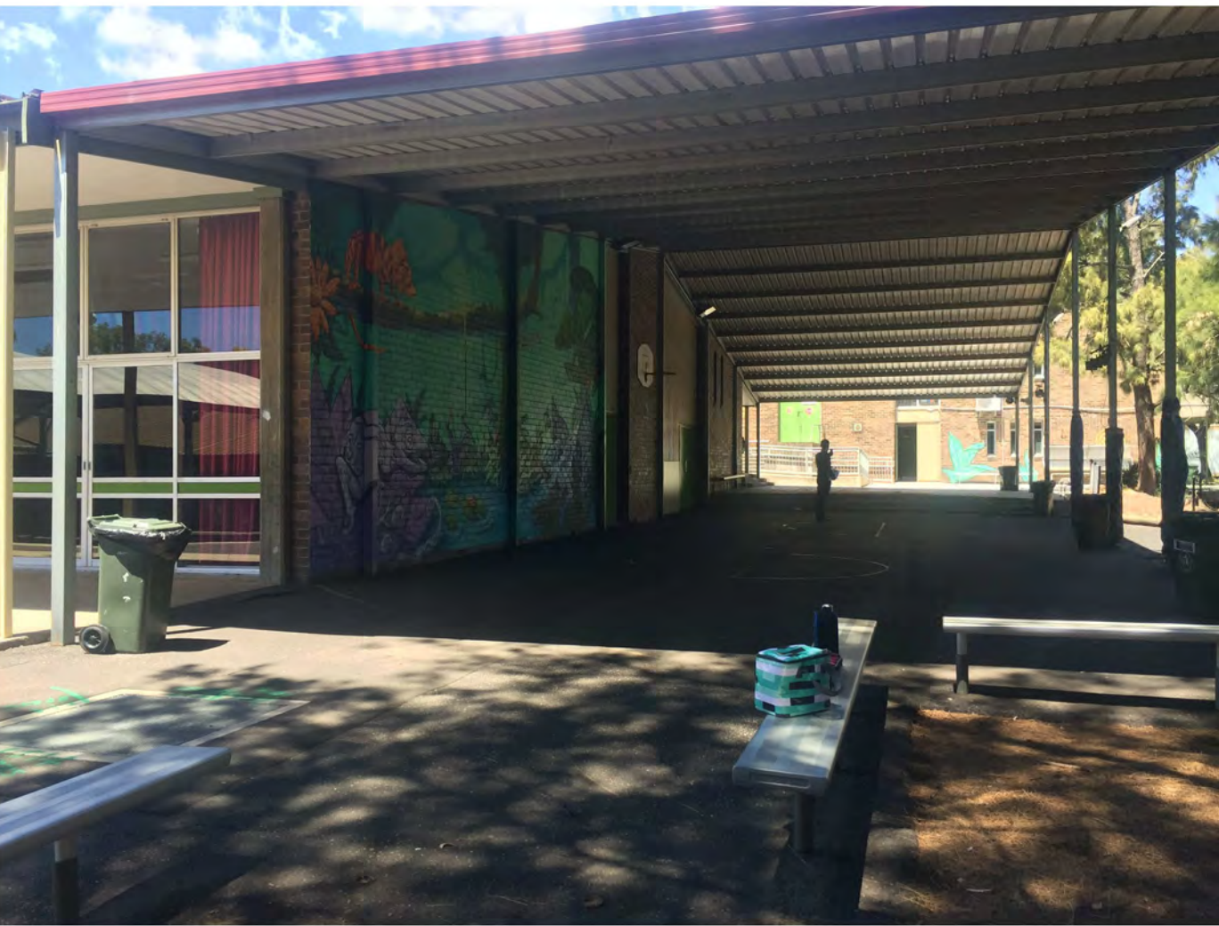
EXISTING HALL BUILDING ON SITE
